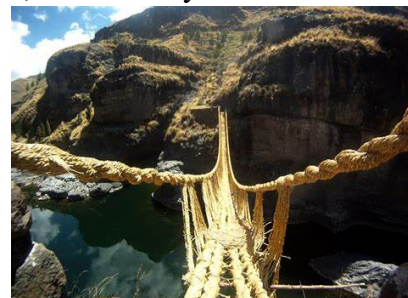
An example of a recently constructed fiber bridge using the Incan technique.
